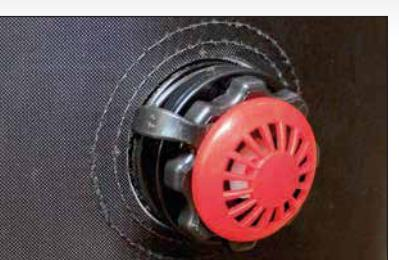
The red Overpressure Valves open automatically as soon as the Bladder is properly pressurized. To test them, unscrew the housing and make sure that the spring inside the valve can be pushed in. Tightly close each valve after testing.
