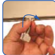
Twist the spring clip to secure to the beam
