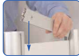
Slide the top beam over the infill panels
