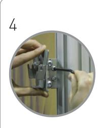
Adjust and tighten 4 screws at side of Interface bracket until securely clamped to post in desired position.
